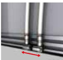
The flexible Zehnder EasyTube connections are ideal for refurbishments too.
